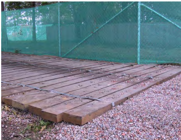
Figure 90- Where access is required through an identified tree protection zone the ground surface shall be protected through appropriate boarding and mulch or gravel placed above the existing ground surface to protect the roots and limit soil compaction. (Photo: Arterra)
