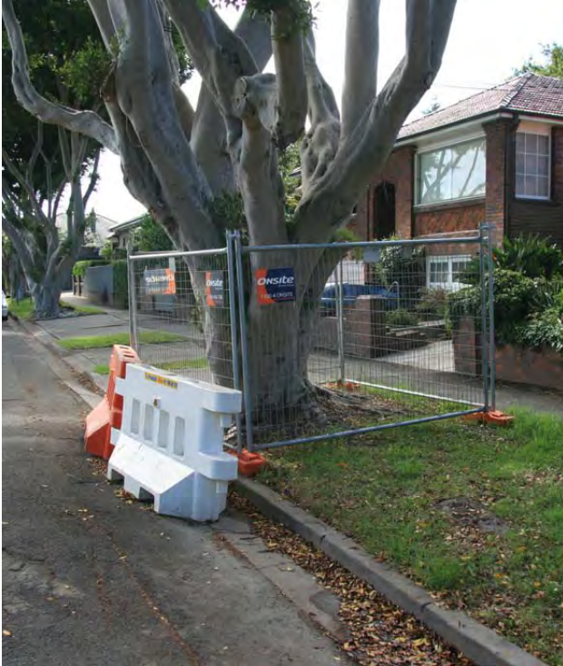
Figure 93- Where tree trunks are low branching and difficult to protect with other methods, water filled barricades and fencing may also be applied. (Photo: Arterra)
