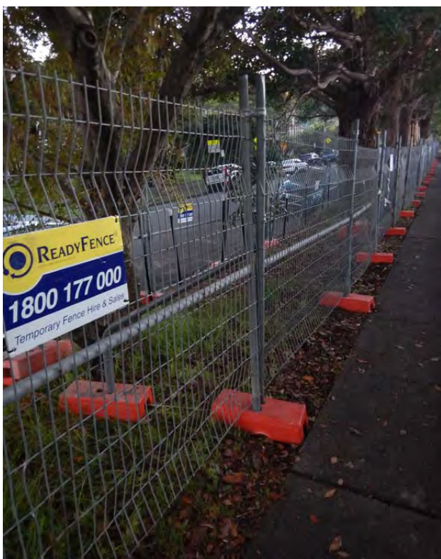
Figure 91- Groups of street trees within a grass strip may also require tree protection fencing installed to protect the trees and the ground surface around them. (Photo: Arterra)
