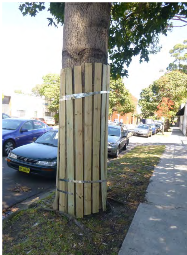
Figure 89- This illustrates the minimum trunk protection measures expected by the Council for street trees adjoining construction sites. (Photo: Arterra)
