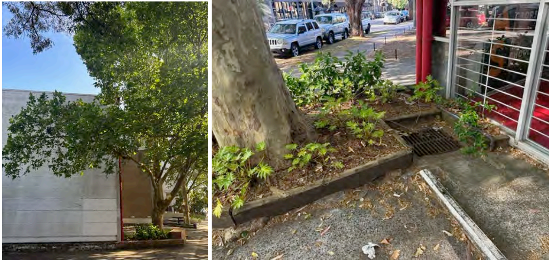
Figures 46 & 47: The proximity of Tree 4 to the existing building edge (Left) and the slab and drain between the trunk and the building(Right). (Source: Austin 2 nd November 2023)
